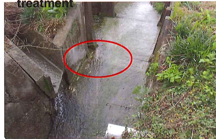
Waterway situation after treatment
