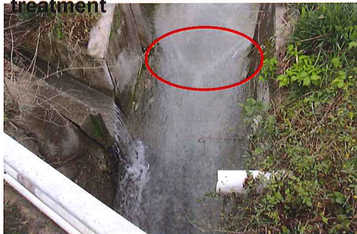
Waterway situation before treatment
